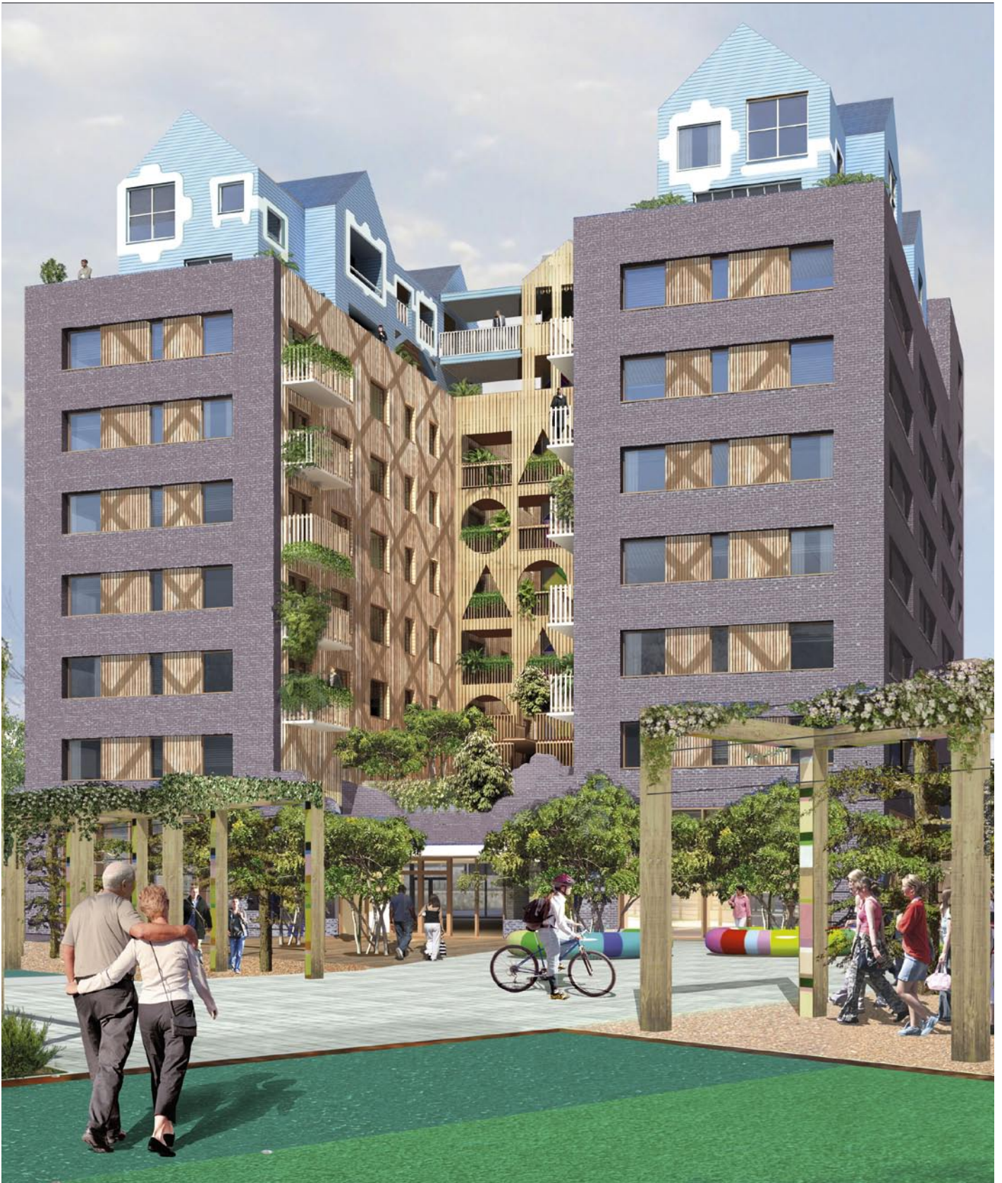
3. The main block will have a brick-dressed concrete frame, with patterned wood cladding around the courtyard
